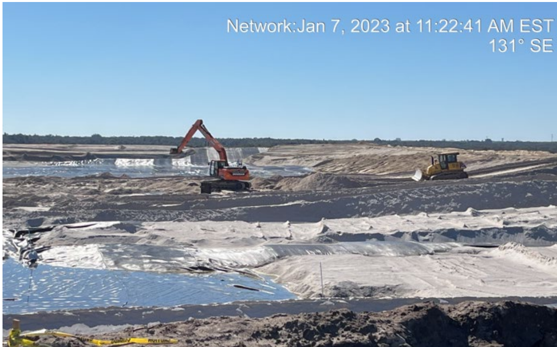
Photo #5 – Dozer pushing sand tailings to long reach.
