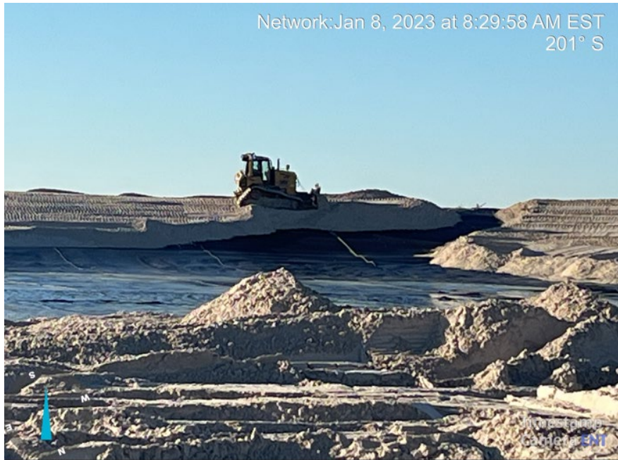
Photo #3 – Sand tailings placement on the south dike using a dozer.
