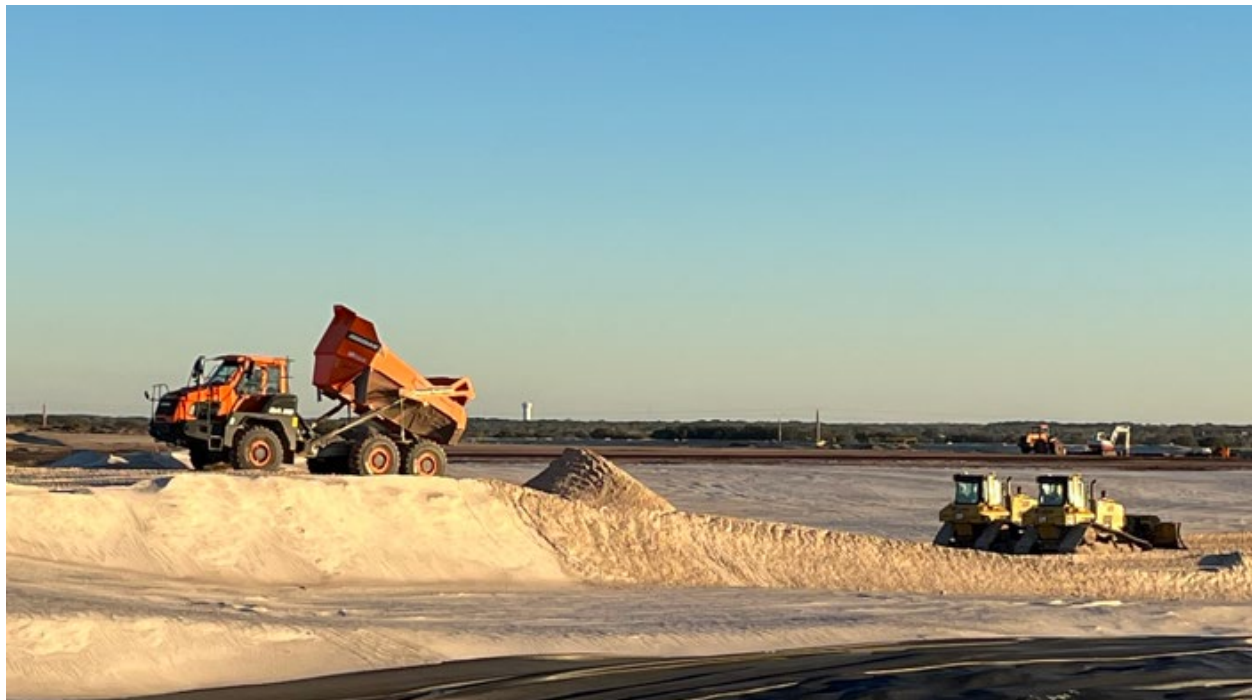
Photo #6 – Dozers placing sand tailings hauled by truck.
