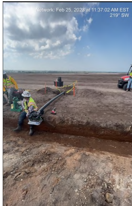
Picture #1 – Installation of gas vent.
