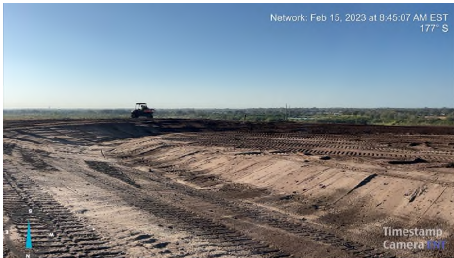
Picture #2 – Subgrade preparation for liner installation.
