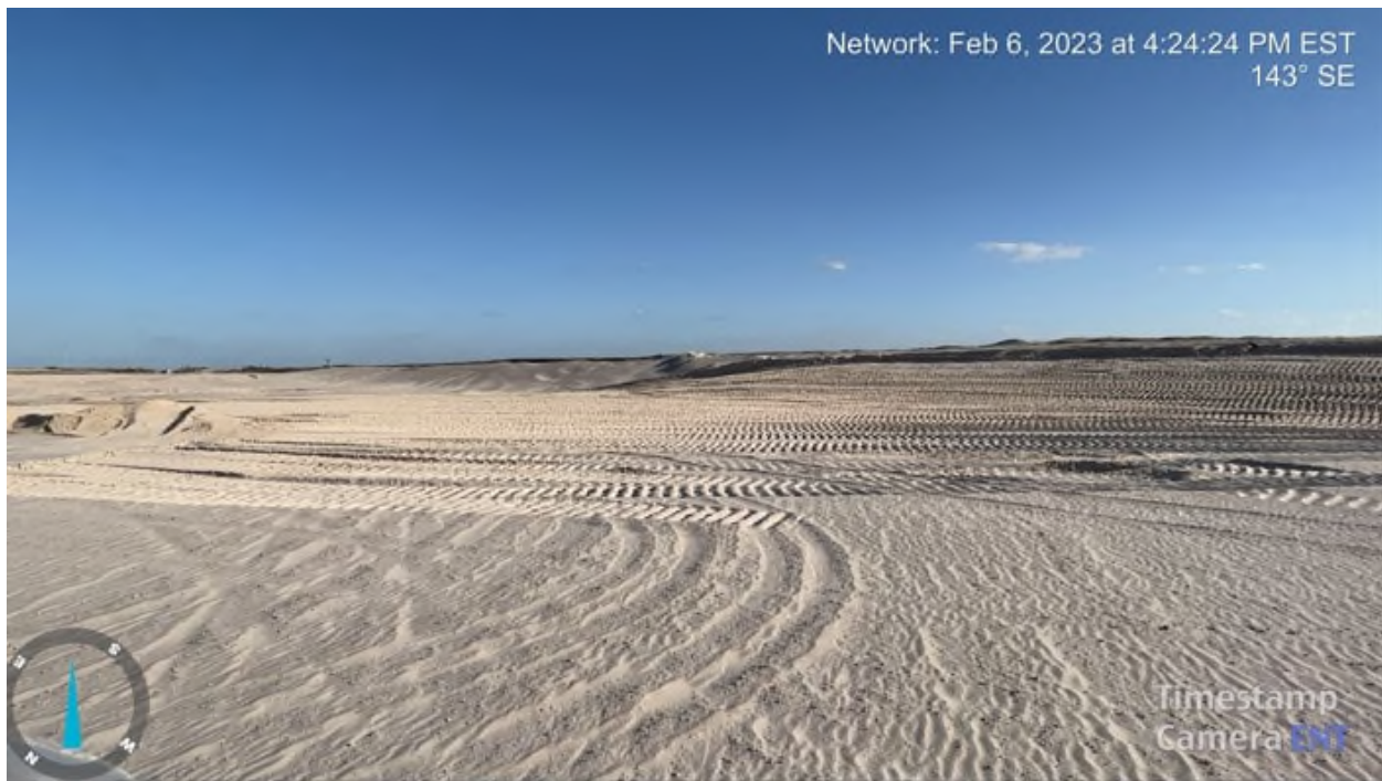
Picture #4 – Progress of sand tailings placement.
