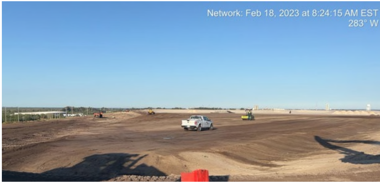
Picture #3 – Subgrade preparation for liner installation.
