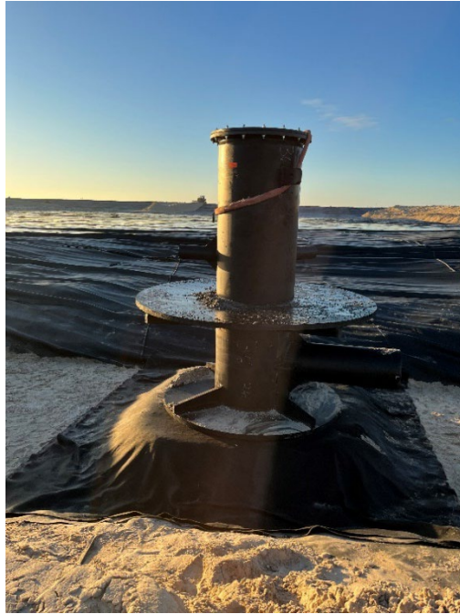
Picture #1 - 36" stormwater inlet structure in place.
