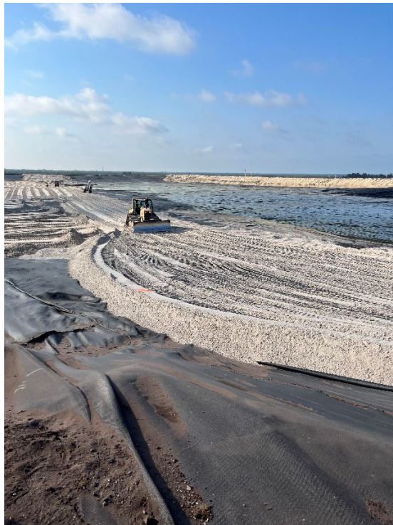
Picture #4 - Constructing the pinch dike.
