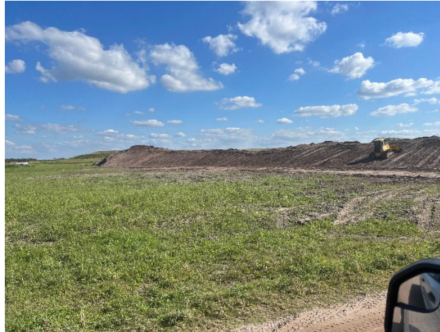
Picture #3 - Maintaining the soil stockpile.
