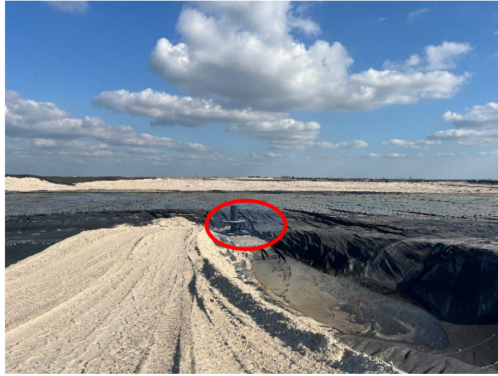
Picture #5 - Sand placement by the 36" stormwater inlet structure.
