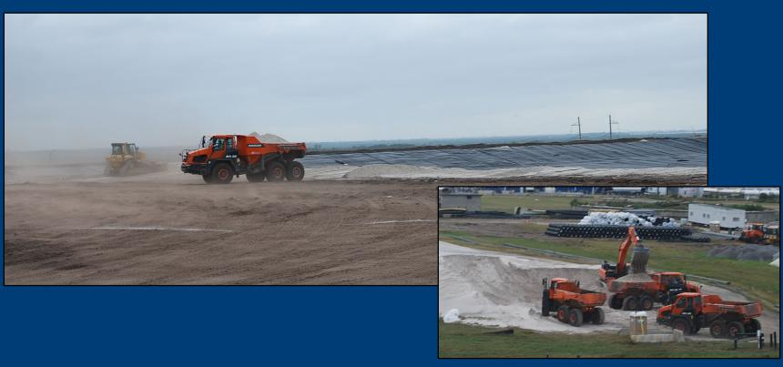
View of ongoing work for the OGS-S with placement of clean/graded drainage sand for the drain system layer over geotextile reinforcement fabric, prior to additional fill, grading, and compaction ahead of the new liner installation.
