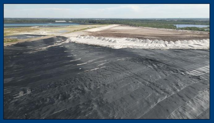
Subgrade reinforcement geotextile deployed over ~ 18 acres inside the OGS-S, as part of the construction of the new OGS-S cap consistent with the Stormwater Management Plan.
