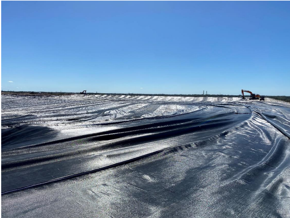
Photo 7 – Deployment the Woven High-Strength Fabric
