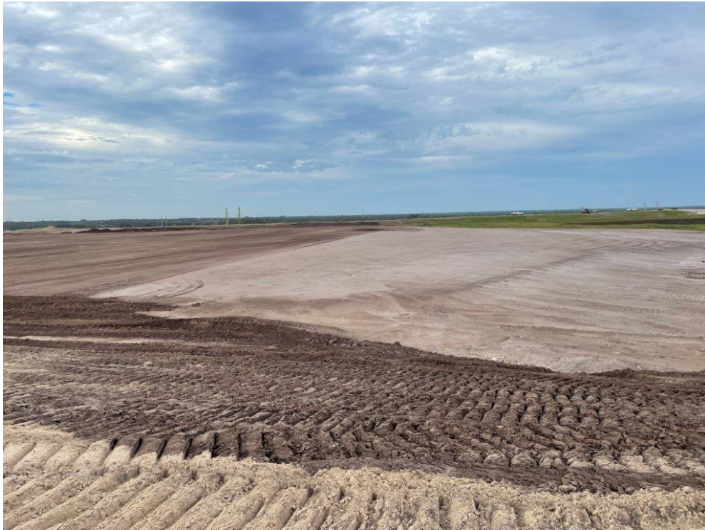
Photo 11 – Completed Placing and Compacting 1-foot Thick Layer of Soil
