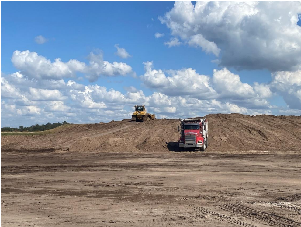
Photo 3 – Fill Material Stockpile
