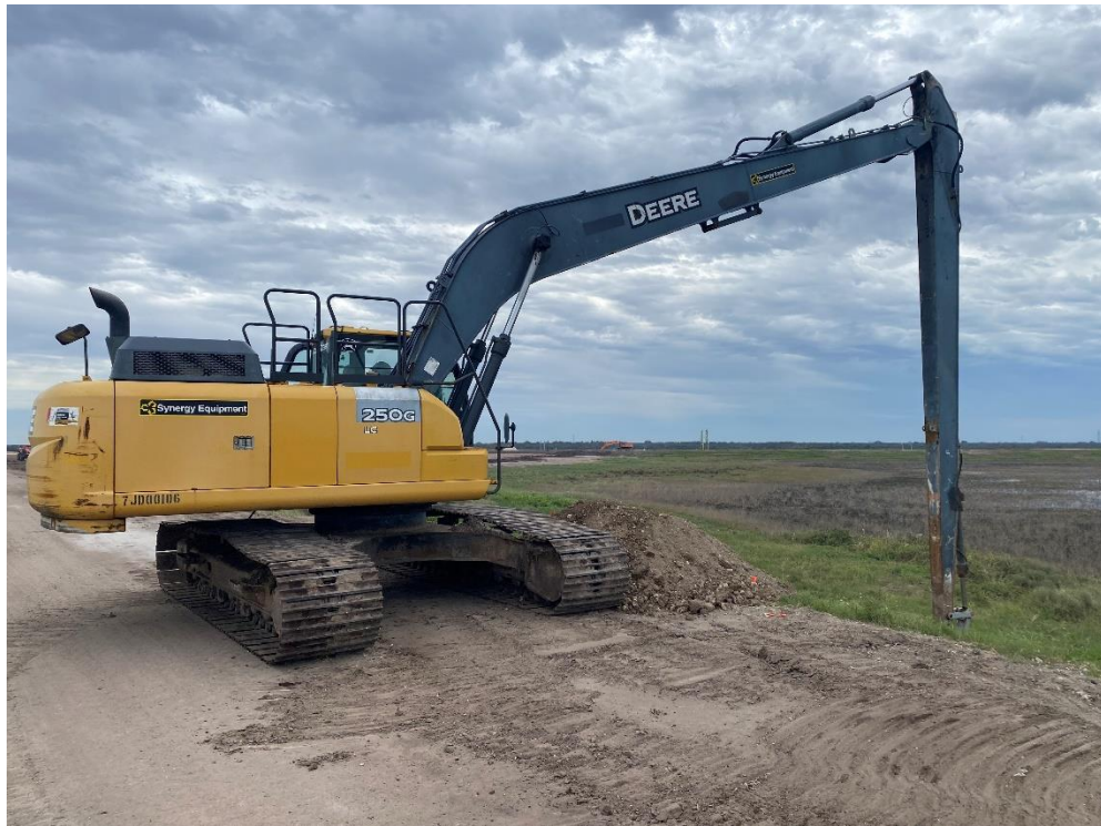
Photo 9 – Locating the Two Existing HDPE Between OGS-S and OGS-N
