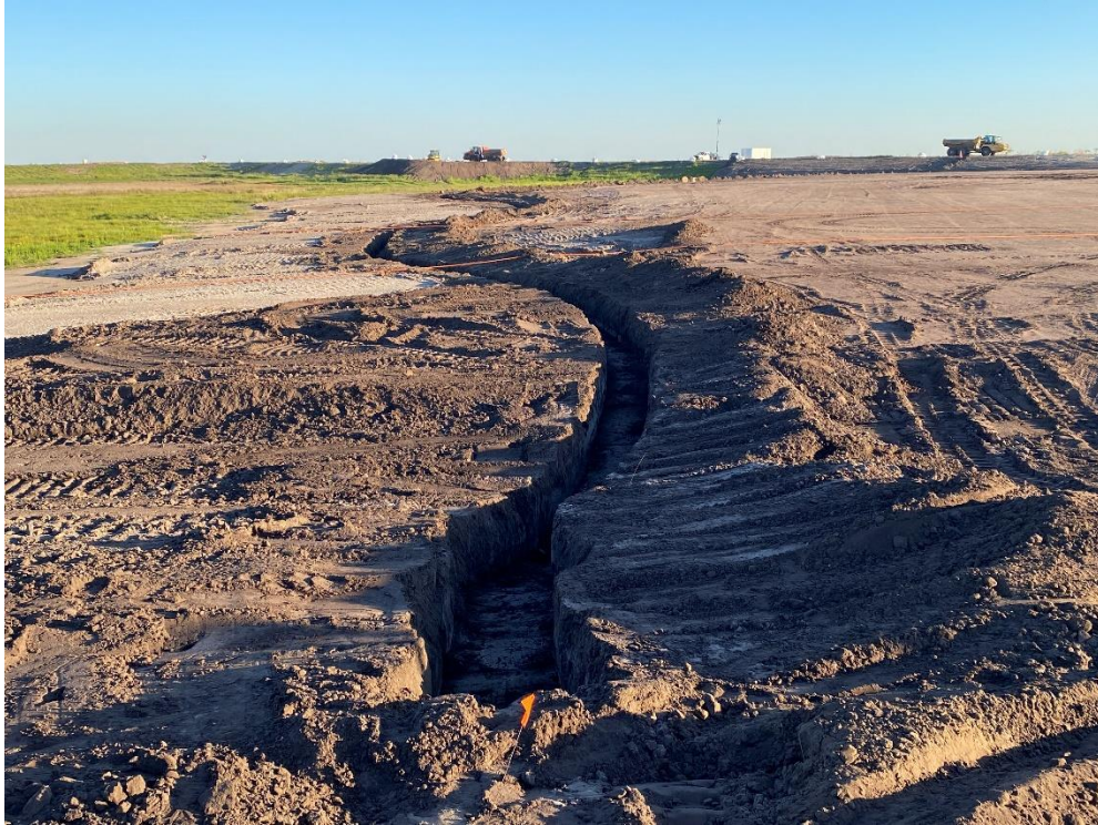
Photo 16 – Anchor Trench for the High-Strength Fabric Installation
