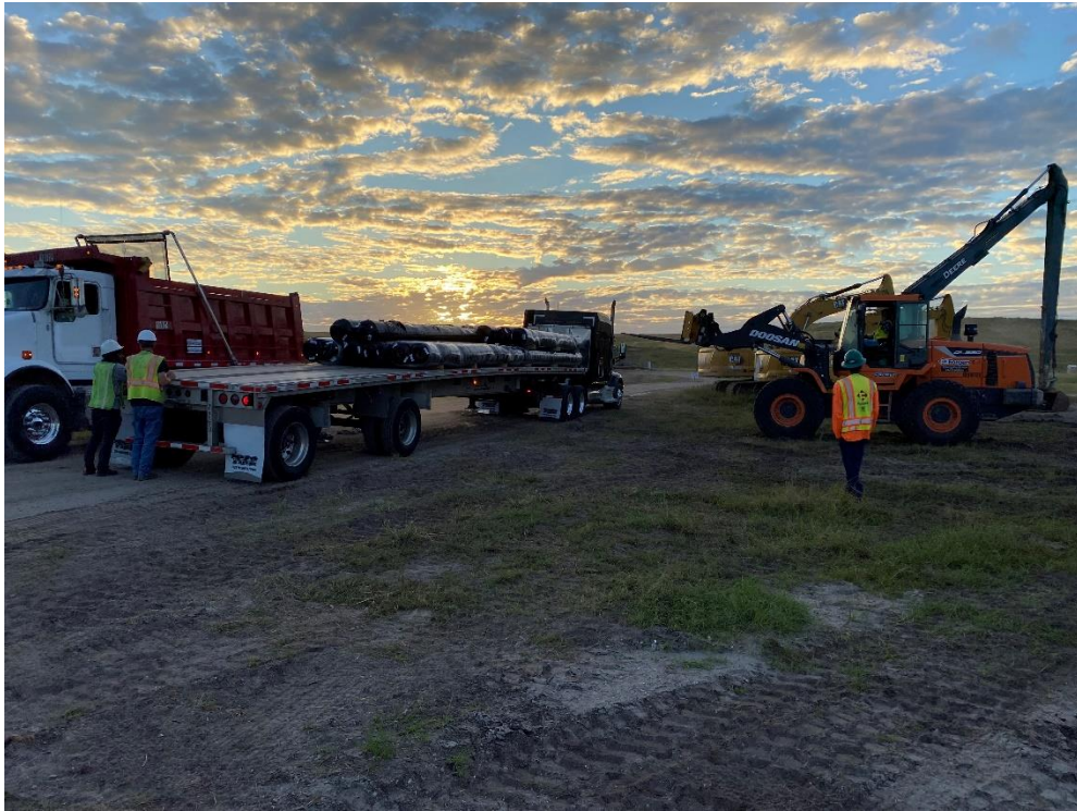
Photo 13 – Material Delivery of Non-Woven Rolls
