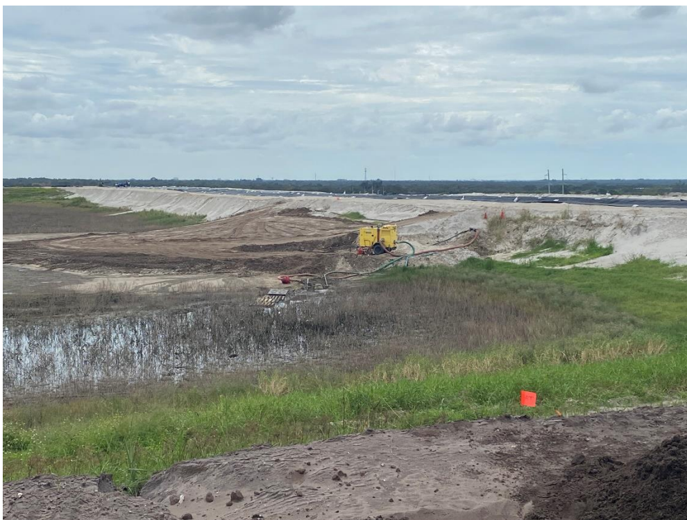
Photo 12 –Dewatering Activities in OGS-S
