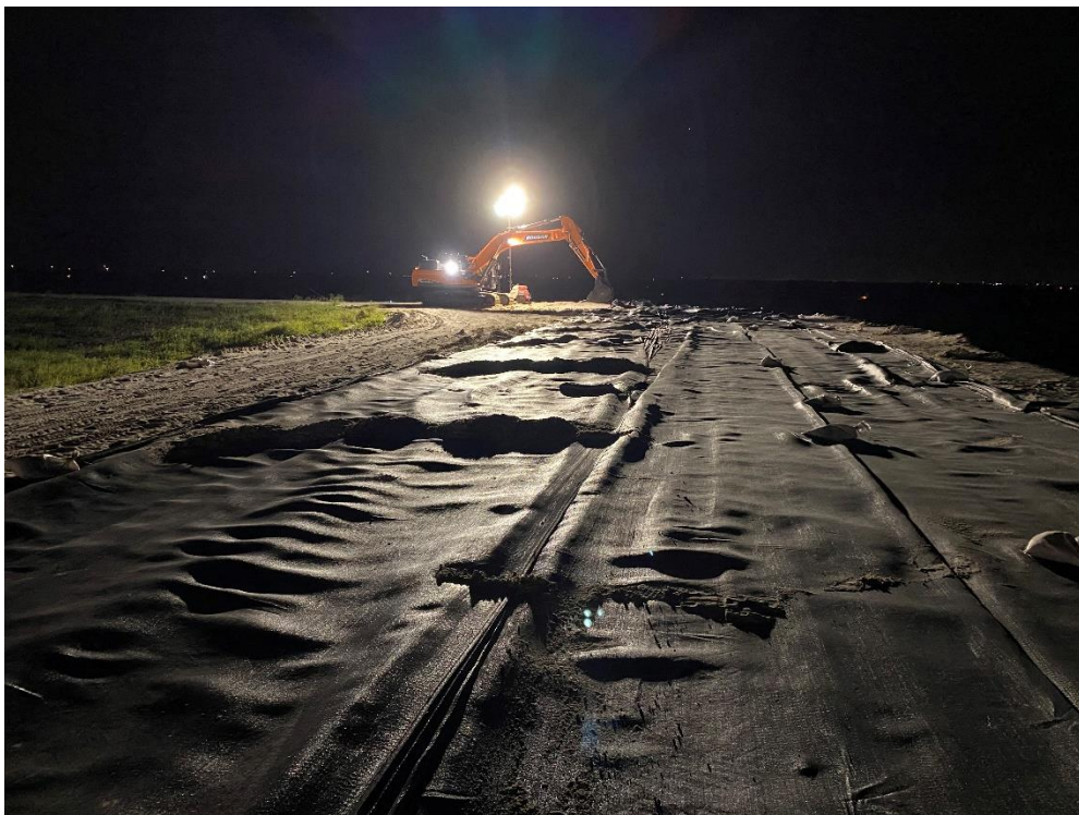
Photo 6 – Started the Deployment of the Woven High-Strength Fabric (5:00 AM)
