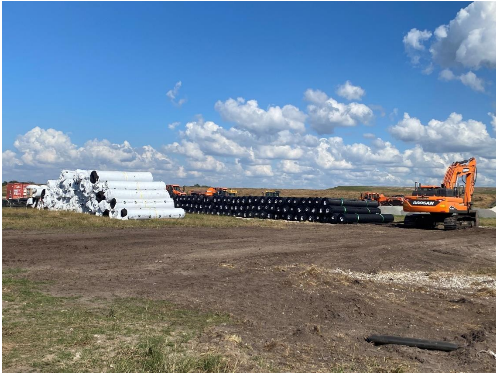
Photo 15 – Staging Area (Liner, Non-Woven Fabric, and Geocomposite)
