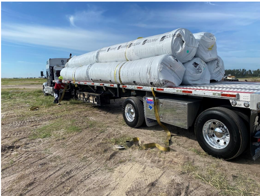
Photo 14 – Material Delivery of Double-Sided Geocomposite Rolls
