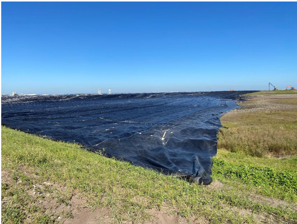
Photo 8 – Deployment the Woven High-Strength Fabric
