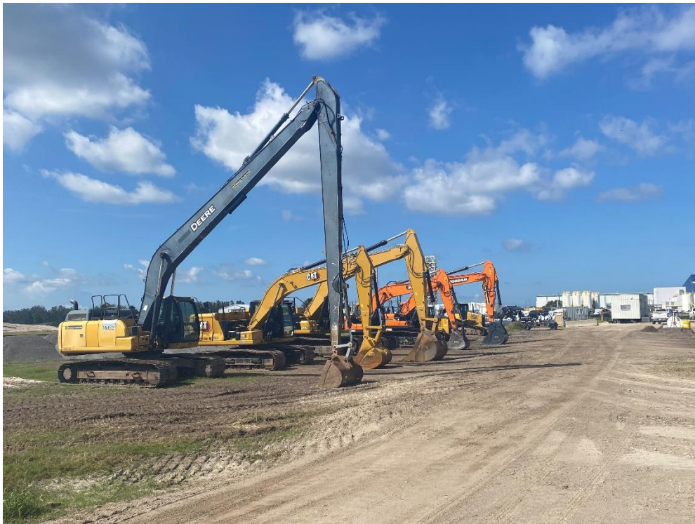
Photo 1 – Construction Equipment in Laydown Area
