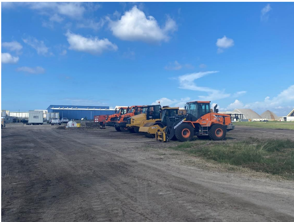
Photo 2 – Construction Equipment in Laydown Area
