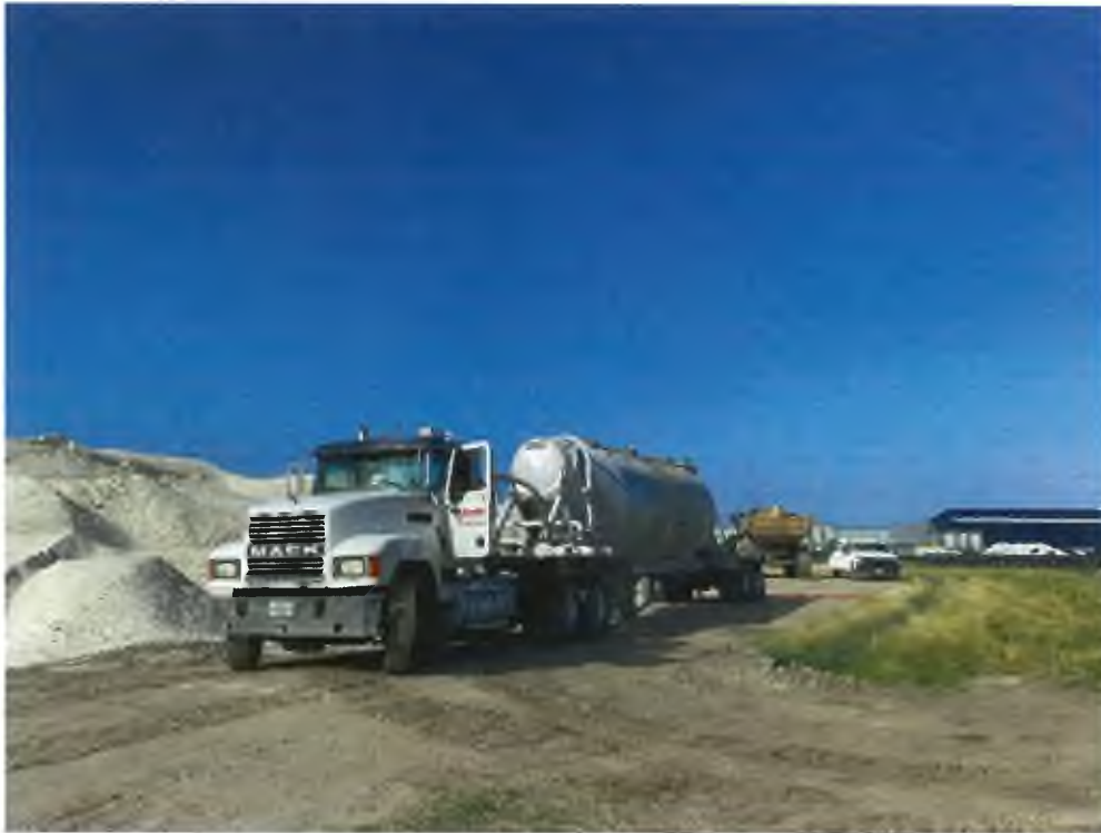
Photo 13 - Received Loads of Portland cement to Perform Bucket Mixing
