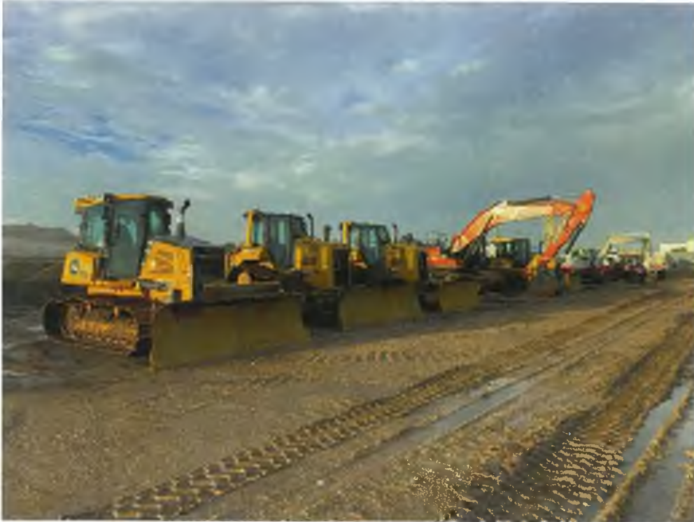
Photo 2 – Construction Equipment in Laydown Area (2)
