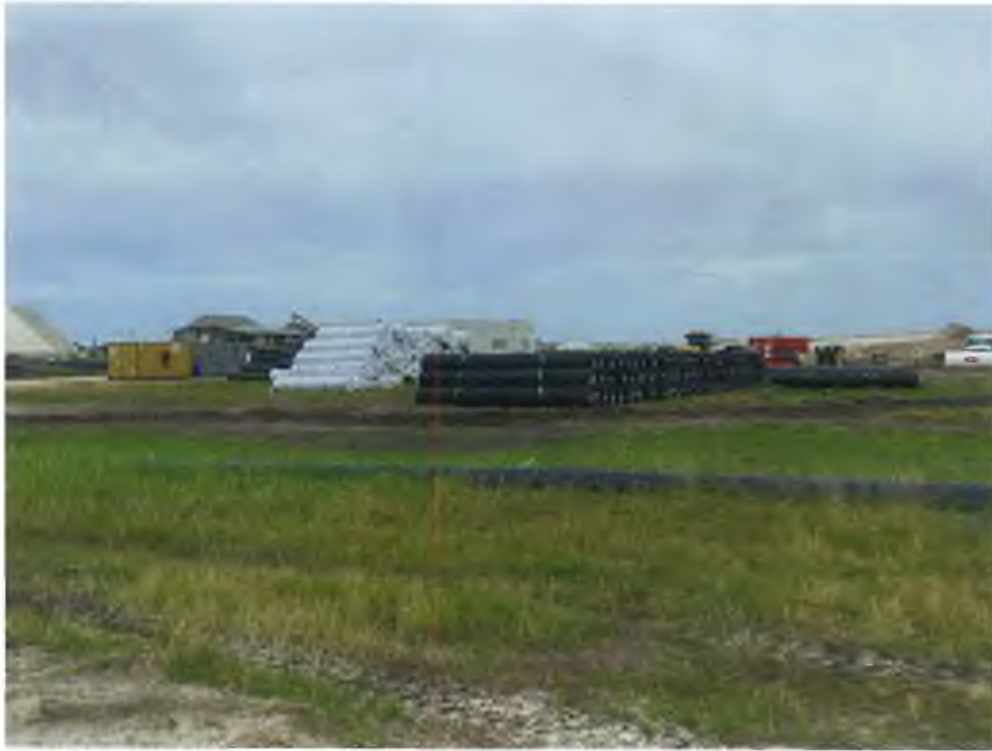
Photo 5 – Staging Area (HDPE Liner, Non-Woven Fabric, and Geocomposite)
