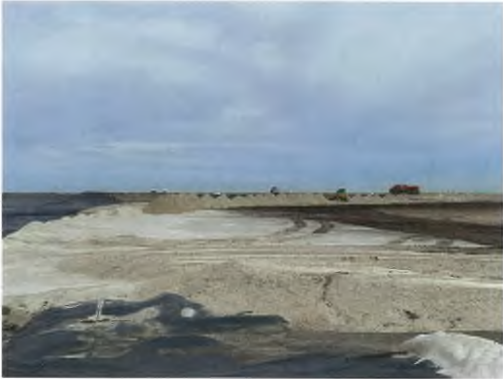
Photo 9 – Placement of Sand Tailings on Top of High Strength Fabric
