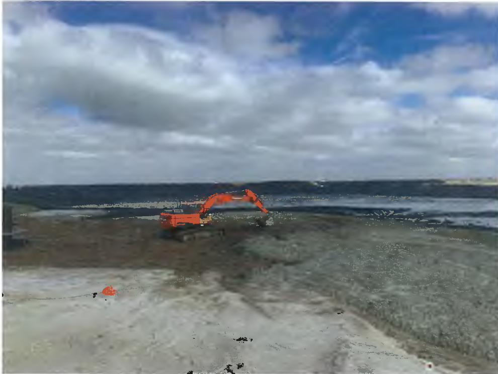
Photo 14 - Bucket Mixing the Sump Area with Portland Cement
