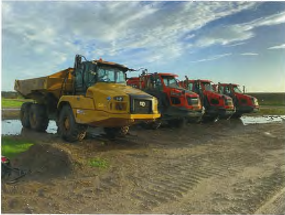
Photo 1 – Construction Equipment in Laydown Area (1)
