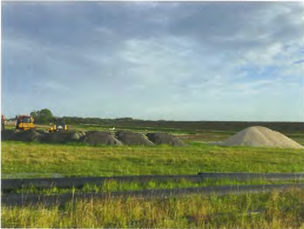
Photo 4 – Stockpile of #7 Gravel and #57 Gravel
