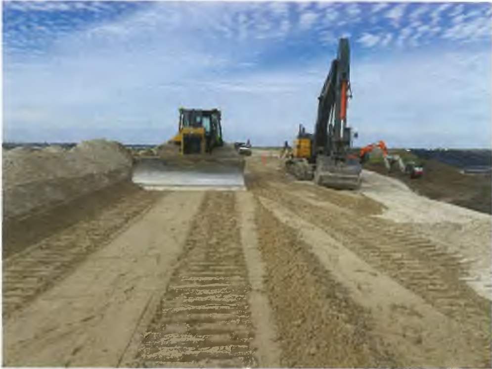
Photo 10 - Grading the Western Dike and Excavating the West Anchor Trench
