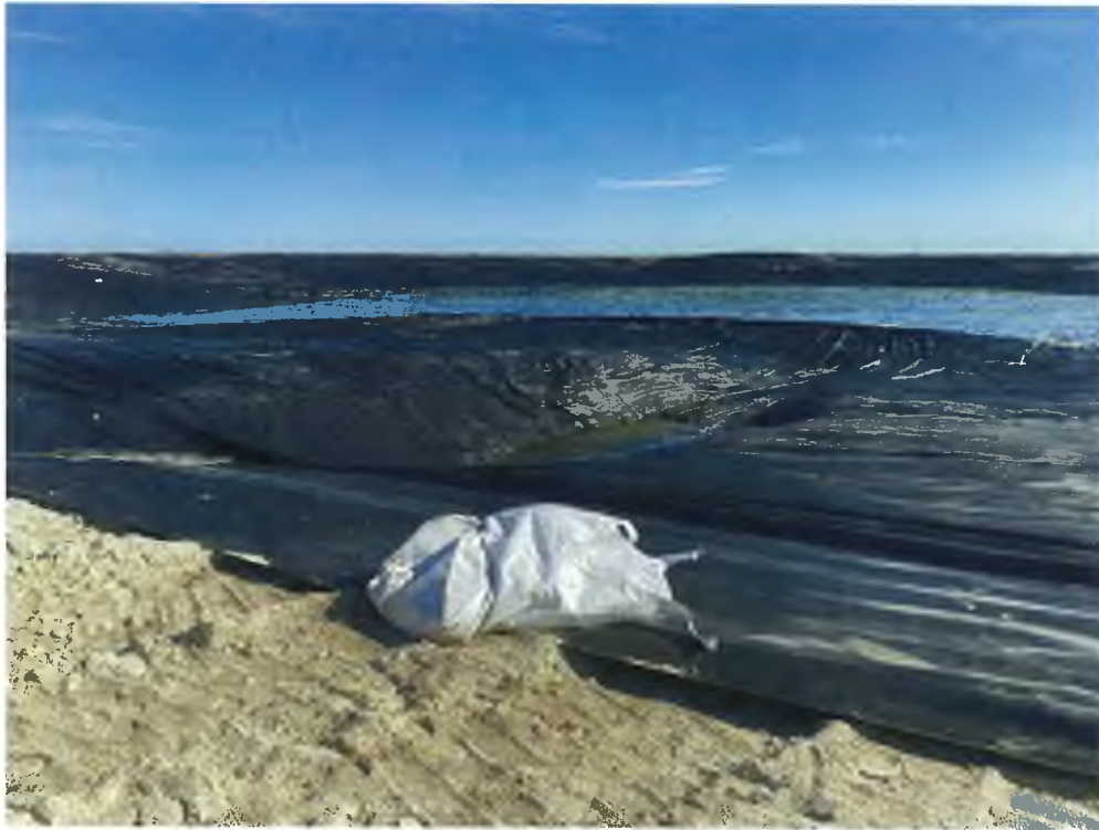
Photo 19 – Soft Sediment Area after Placement of High-Strength Fabric (2)
