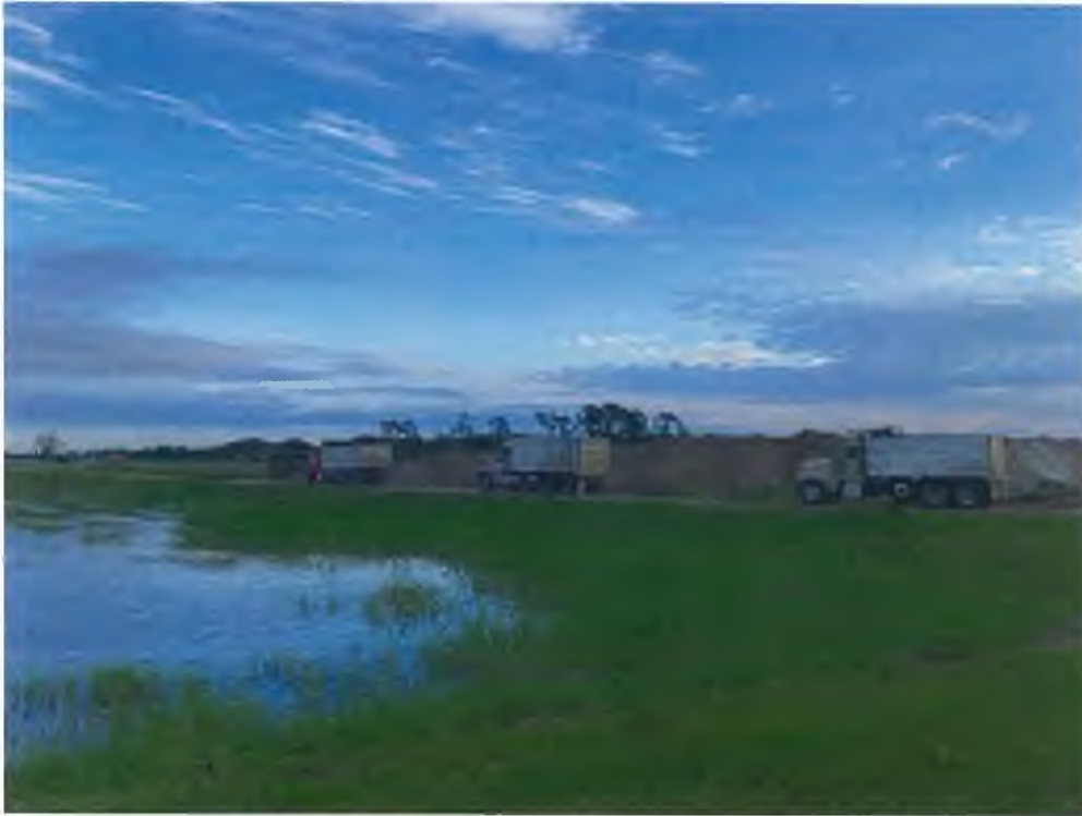
Photo 3 – Haul Trucks Delivering Soil Fill and Sand Tailings
