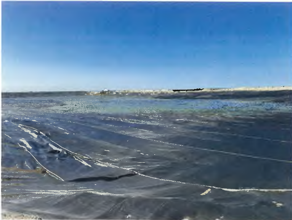
Photo 18 – Soft Sediment Area after Placement of High-Strength Fabric (1)
