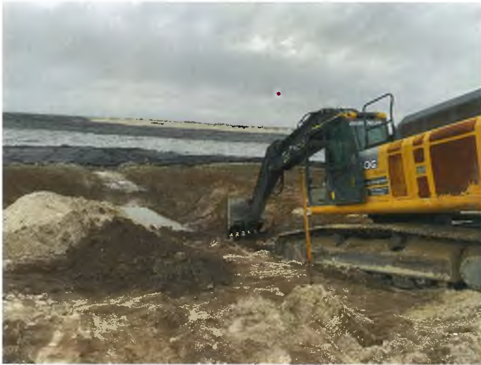
Photo 15 – Excavation of the Outlet Structure
