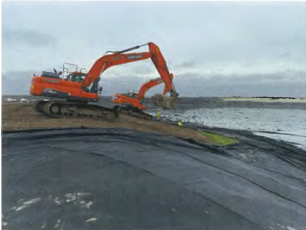
Photo 16 - Deployment of the High-Strength Fabric
