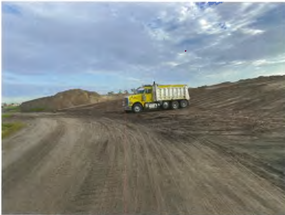
Photo 6 – Soil Fill Material Stockpile
