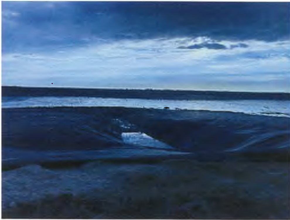
Photo 17 – Placement of High-Strength Fabric Inside the Excavated Sump Area
