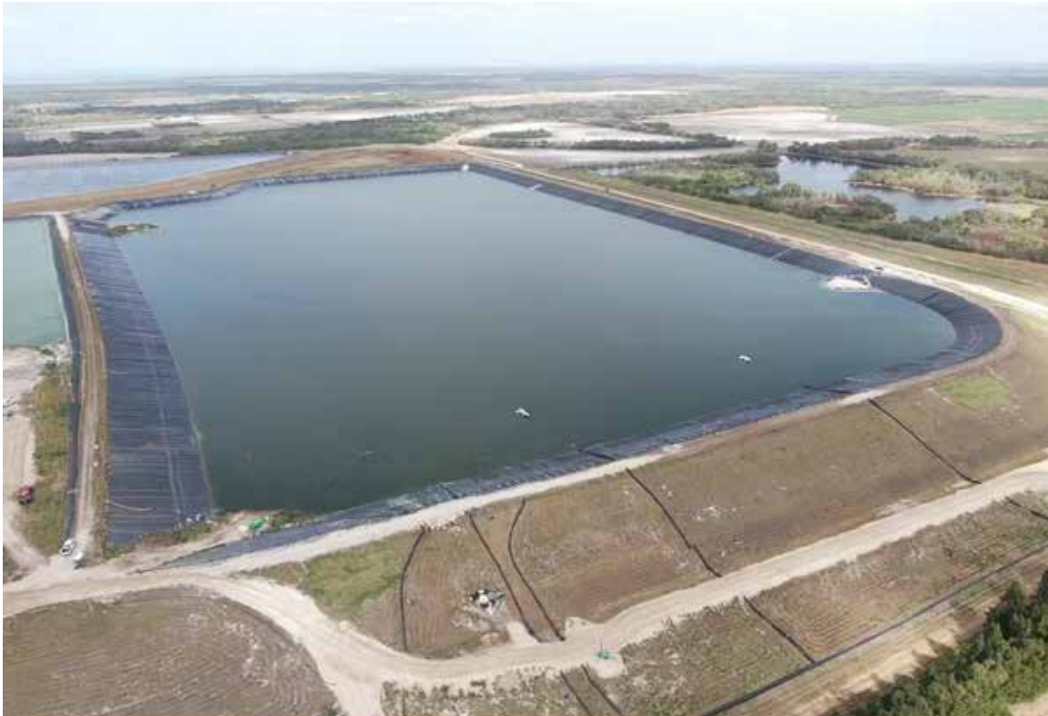
Picture of New Gyp Stack South (NGS-S) courtesy of Garner Environmental Services, Inc.
