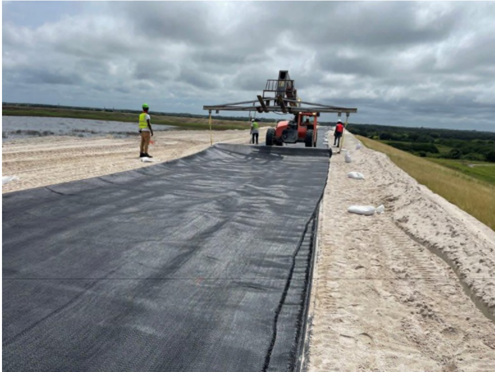
Photo 2 – Deploying the Woven High-Strength Fabric
