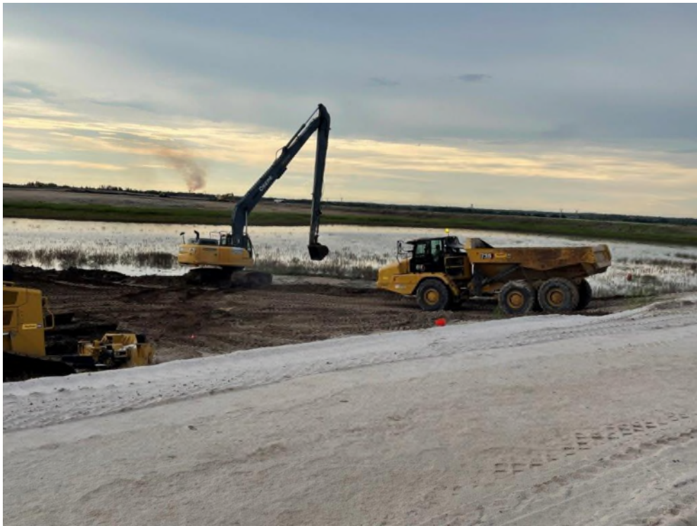
Photo 15 – Excavating and Grading the Sump Area
