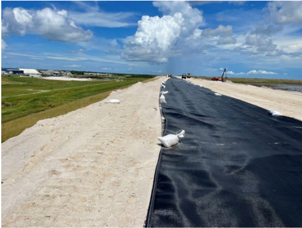
Photo 1 –Placing the Woven High-Strength Fabric
