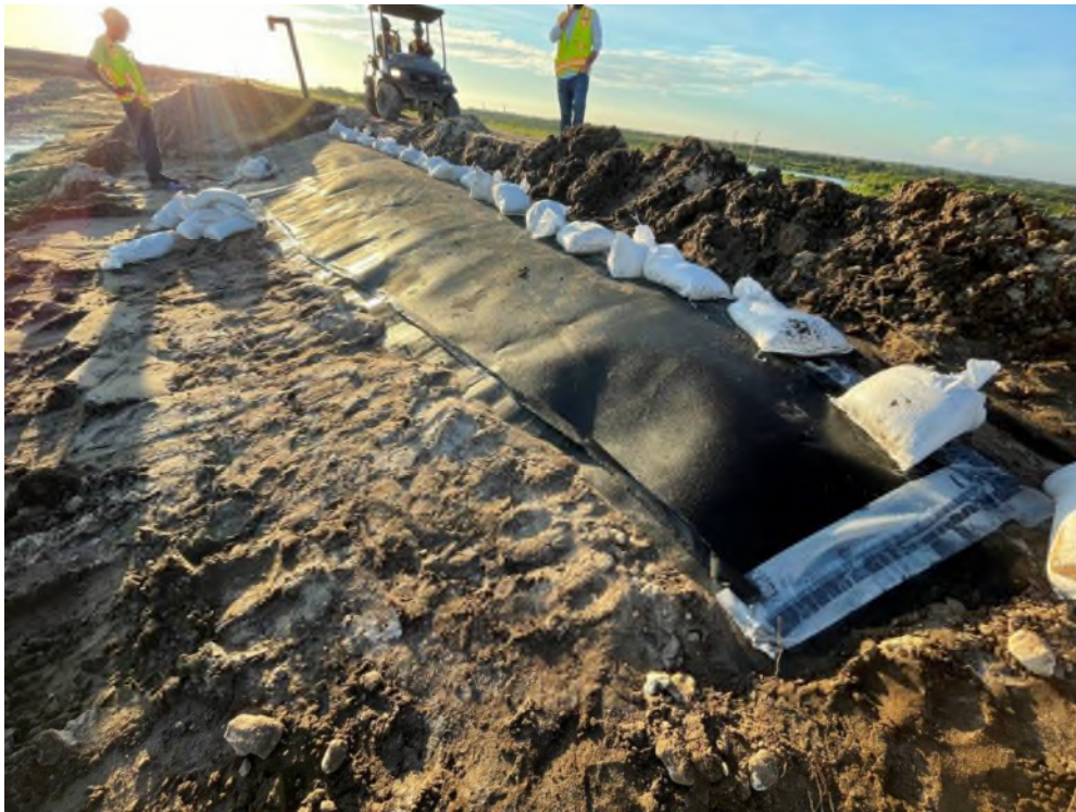
Photo 13 – Temporary Repair of the Primary Liner Tear
