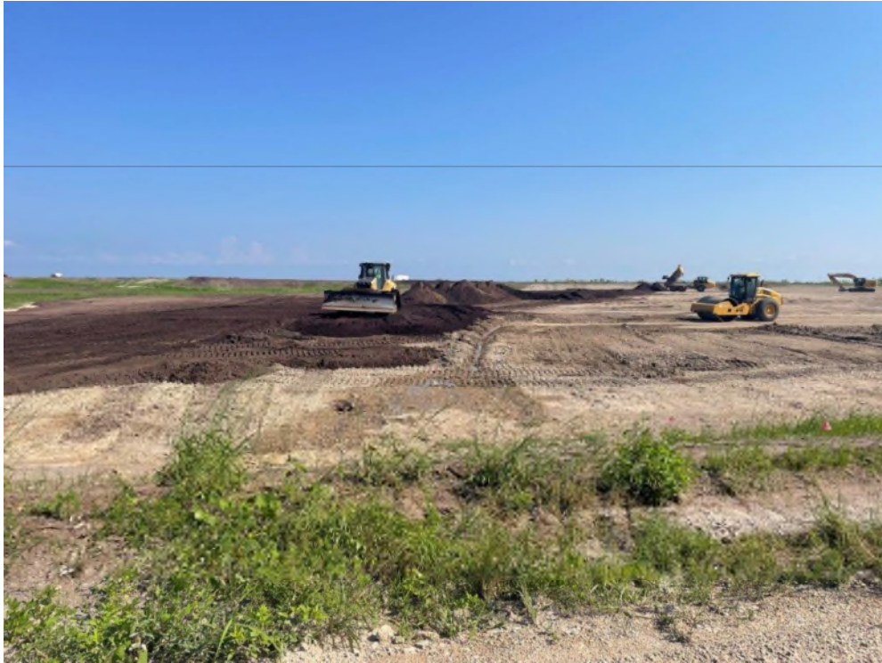
Photo 12 – Placement and Compaction of a 1-foot Thick Layer of Soil
