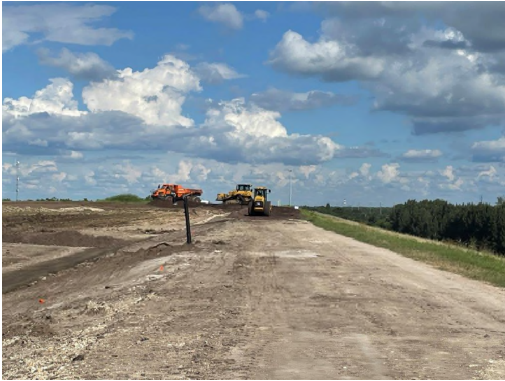
Photo 11 – Placement and Compaction of a 1-foot Thick Layer of Soil
