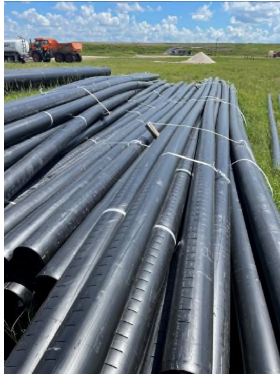
Photo 6 – Welding the Slotted 6-inch HDPE Pipes
