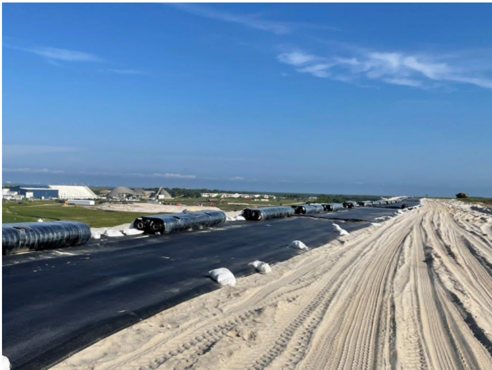
Photo 16 - Site Preparation for Hurricane Ian
