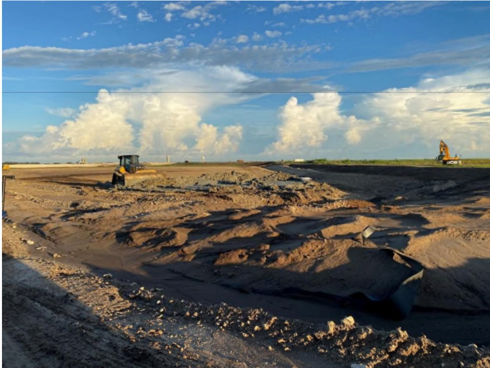
Photo 14 – Completed Exposing the Old Secondary Liner on the East Dike
