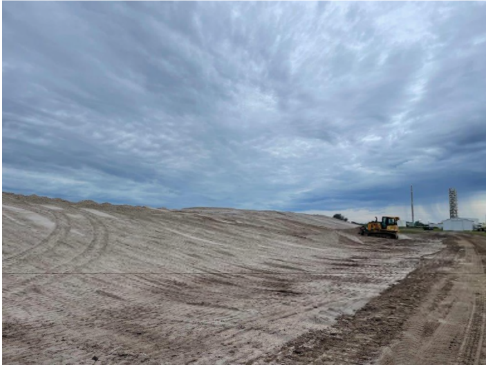
Photo 4 – Sand Tailings Stockpile
