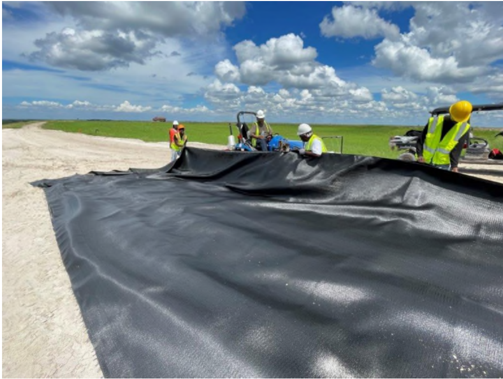
Photo 3 – Sewing the Woven High-Strength Fabric
