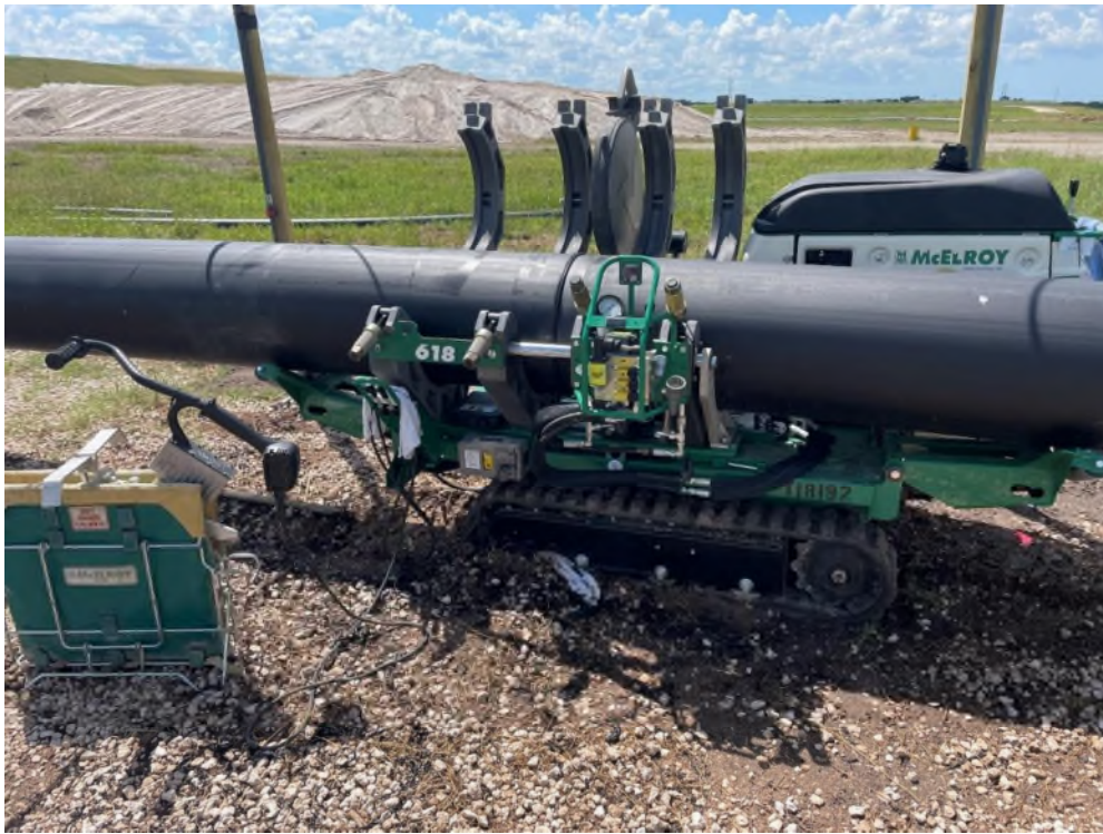
Photo 5 – Welding the 18-inch HDPE pipes
