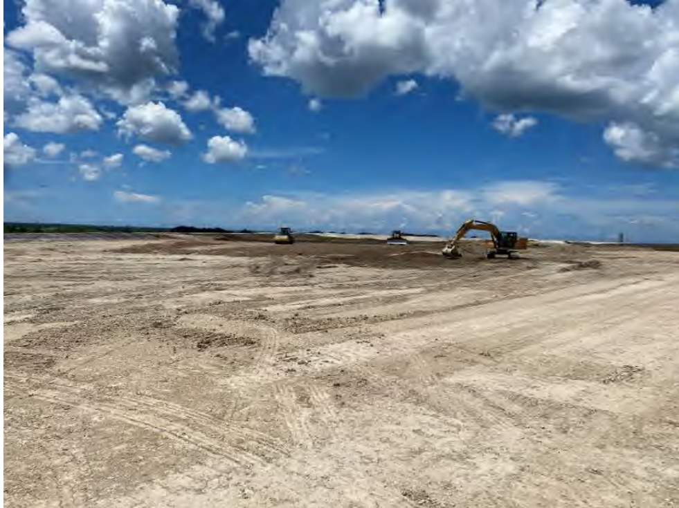
Photo 2 – OGS-S Construction Area
