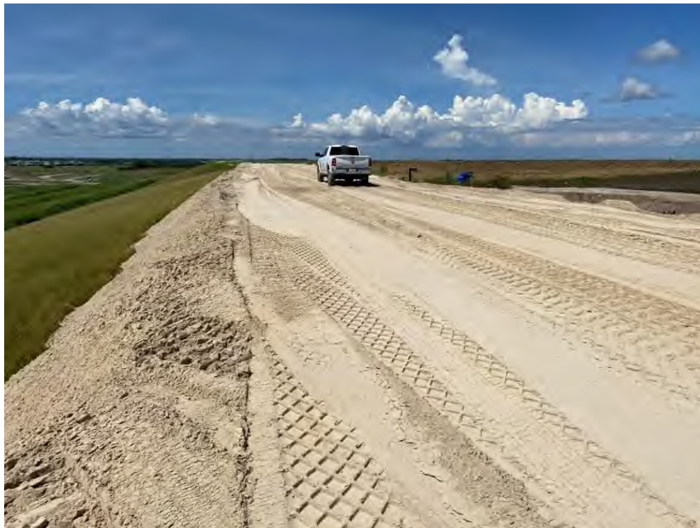
Photo 6 – Widening of West Berm (1)
