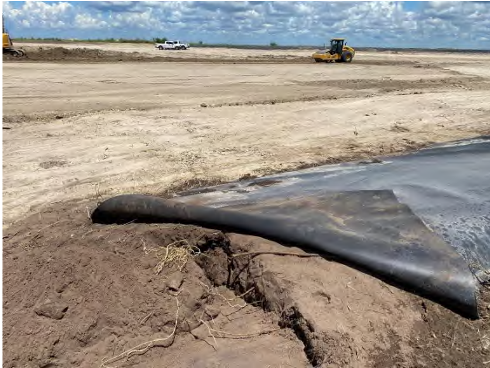
Photo 11 – Exposed the Secondary Liner on the South Dike.
