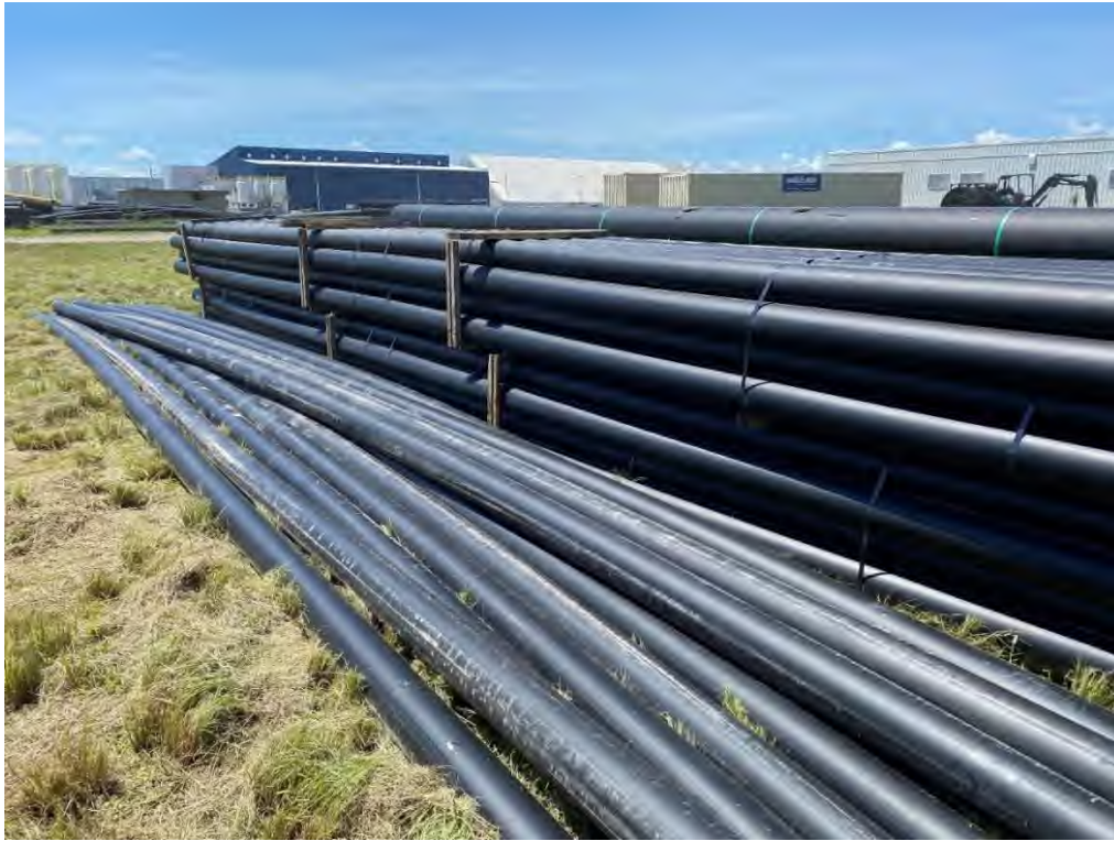
Photo 5 – On-site Storage of Pipes
