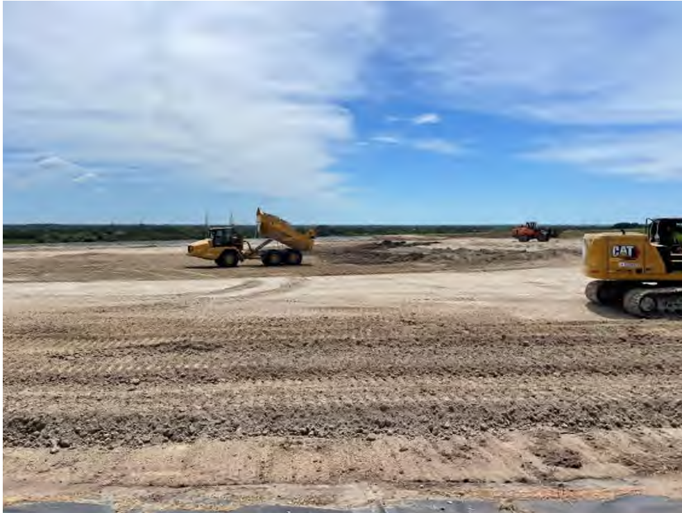
Photo 10 – Graded East Slope Drainage Ditch
