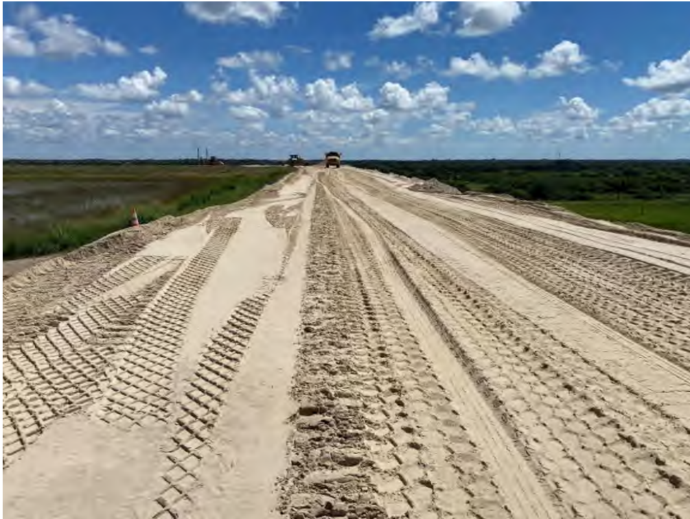
Photo 7 – Widening of West Berm (2)
