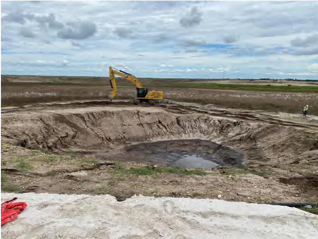
Photo 13 – Started Dewatering and Grading Sump Area
