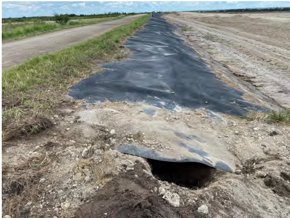
Photo 12 – Exposed the Secondary Liner on the East Dike.
