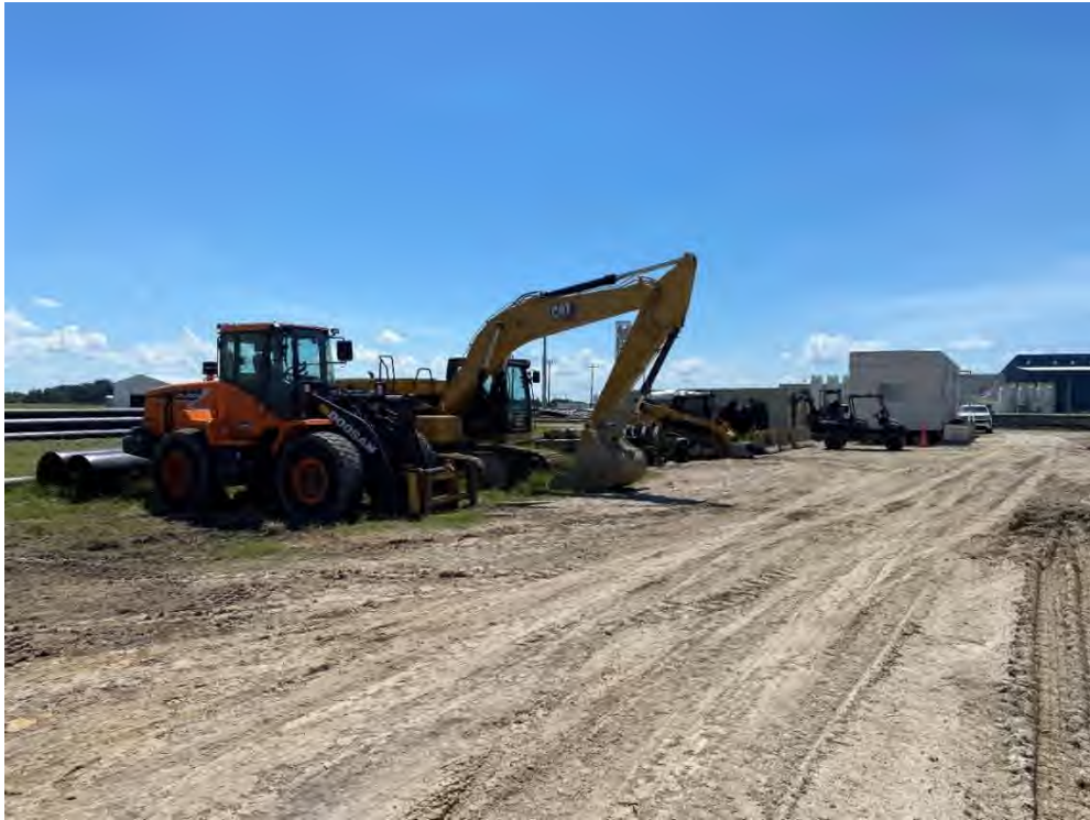
Photo 1 – Construction Equipment in Laydown Area
