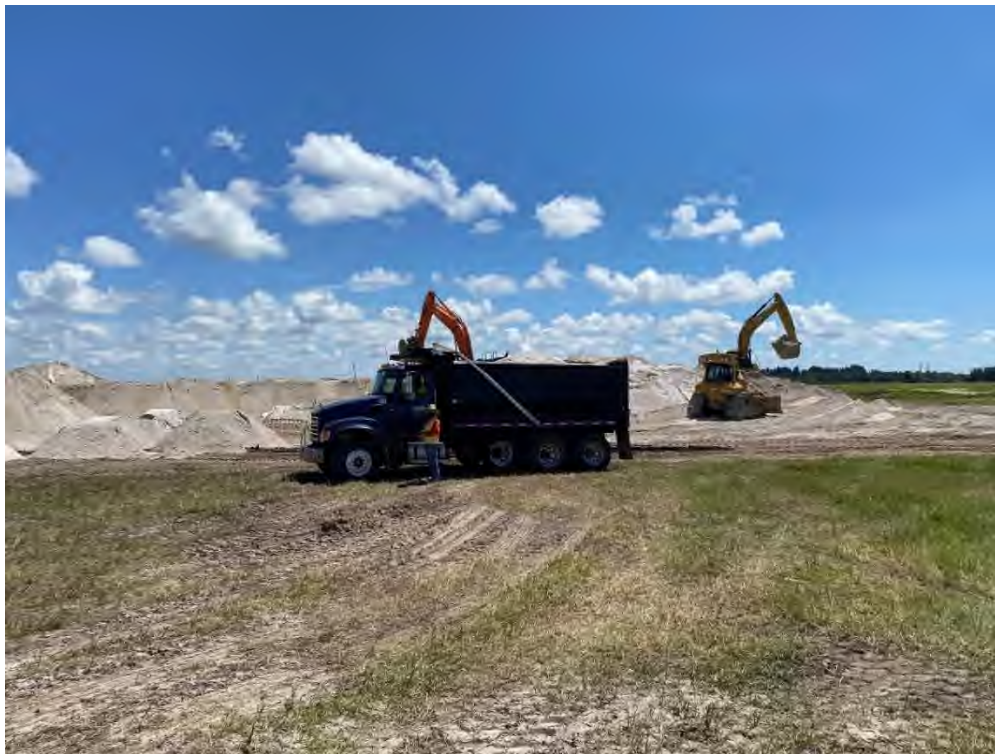
Photo 4 – Sand Tailings Material Delivery
