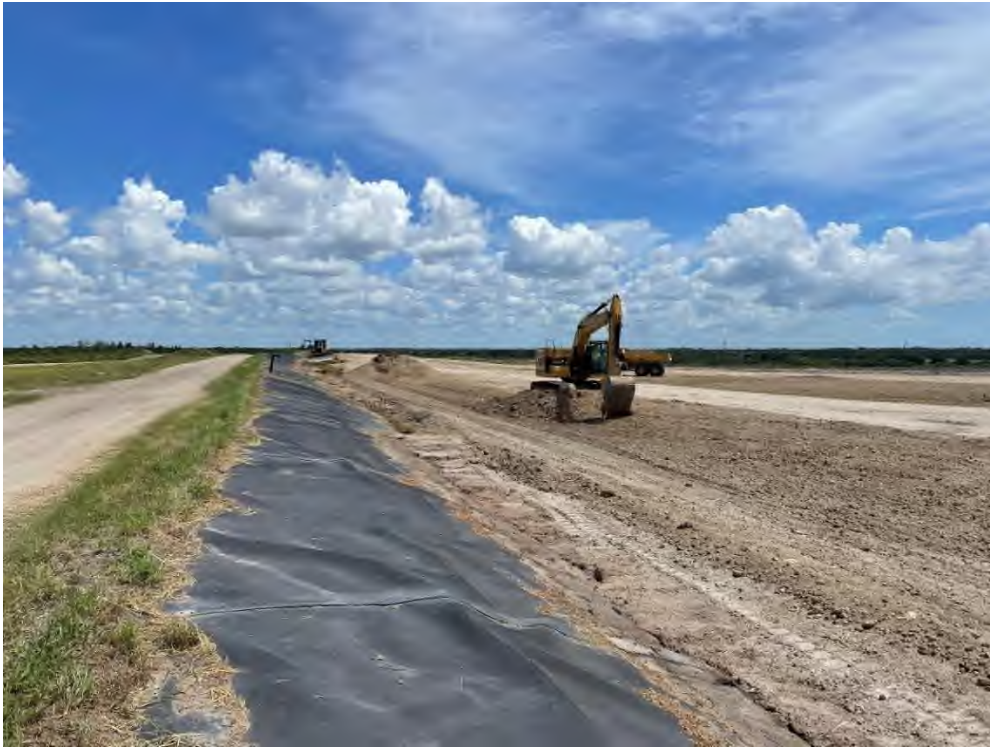
Photo 9 – Grading Coarse Dredge Material on the East Side of OGS-S Pond
